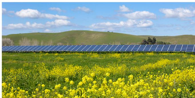
*In 2016, Barr designed a 350 kW solar energy photovoltaic system to work in parallel with four diesel generators on a private island in the British Virgin Islands.*
