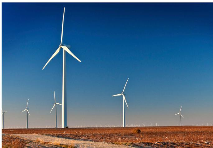
*For a 531-megawatt wind generation facility in Texas, Barr was hired to assist with a project that included over 100 turbines, the associated underground collection system, two 345 kV substations, and 5 miles of transmission line. In addition to designing the project from the ground up, dealing with procurement delays, and adapting to frequent changes in turbine location, our team provided construction support through completion of the project.*
