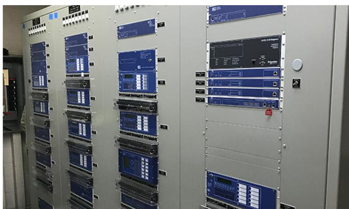
*The Southwestern Power Administration's Poplar Bluff substation included several pieces of equipment in need of upgrading. Barr designed a relay panel to replace outdated protection and controls (P&Cs) and upgraded the remote terminal units (RTUs) and metering equipment.*
